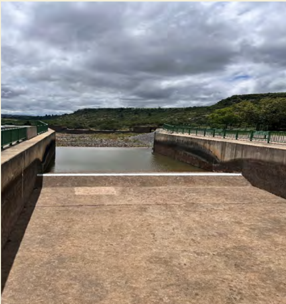
Figure 3: Portion of the Delivery Tunnel (SA side)
