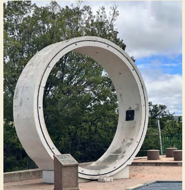
Figure 2: Tunnel section constructed using cement
